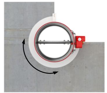
To help you find the suspension plane, a bendable fixing bracket is provided on the damper body (the use of bendable fixing brackets is not required to meet the classification) and the red tape is placed on the casing to mark the location of the wall limit (distance from wall limit to the end of fire damper is 220 mm). This does not apply for Applique/MF1/MF2 kit installations. Check the operation of the fire damper before commencing
